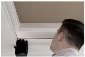
When you see the size is right, the headbox can be taken out again and pre-drilled for easier installation.
