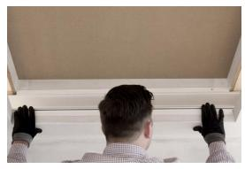
When you see the size is right, the headbox can be taken out again and pre-drilled for easier installation.
