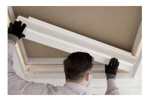
Start by sliding up one end into the recess. Most common installation is to have opening towards the glass and the hinge corner towards the room.
