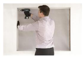
Fix the box using countersink screws through the skim coat flange.
