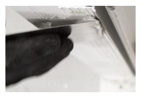
Use skim coat all the way to the chamfered edge.
