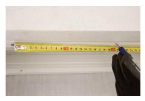
Measure for screws through the skim coat flange at 200mm increments around the box.
