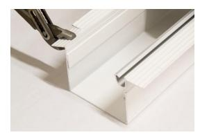
A plier can also be used to wiggle off the flange.
