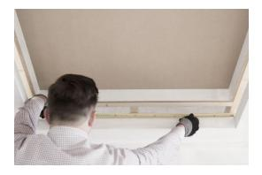
Skylight installation requires precise preparations. Measure all opening lengths and overall recess lengths. Laser can be used.
