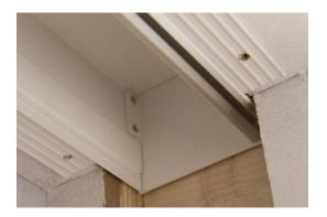
Pre-drilled whole for screw in skim coat flange.
