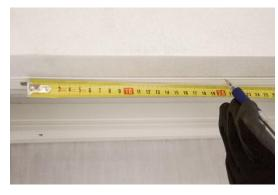
Measure for screws at 200mm increments around the box.
