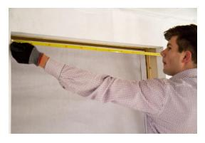
Measure the opening length and the pocket length to allow for end caps and/or side boxes.
