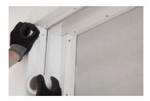
Apply plaster fiber tape of the skim coat flanges.
