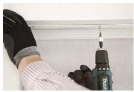
Fix the box with countersink screws at the marks.
