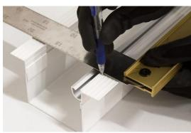
Use a square and mark lines on the skim coat flanges for cutting.
