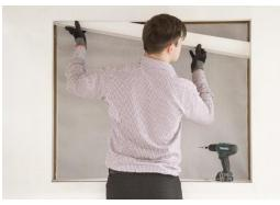
When you see the size is right, the headbox can be taken out again and pre-drilled for easier installation.
