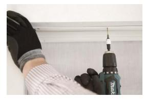
Fix each box with countersink screws at the marks.
