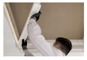
Start by sliding up one end into the recess. Most common installation is to have opening towards the glass and the hinge corner towards the room.
