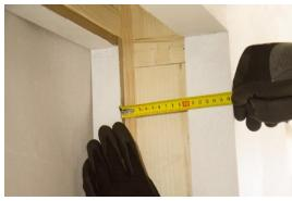
Measure the pocket size at each end and the center where a box will be mounted.
