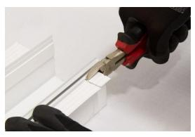
An alternative is using a cutter or saw, to cut away the flange.
